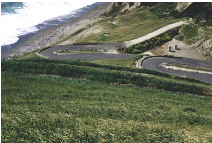
Avalon Canyon Slide Repair – March 1999 – Quick Cover
