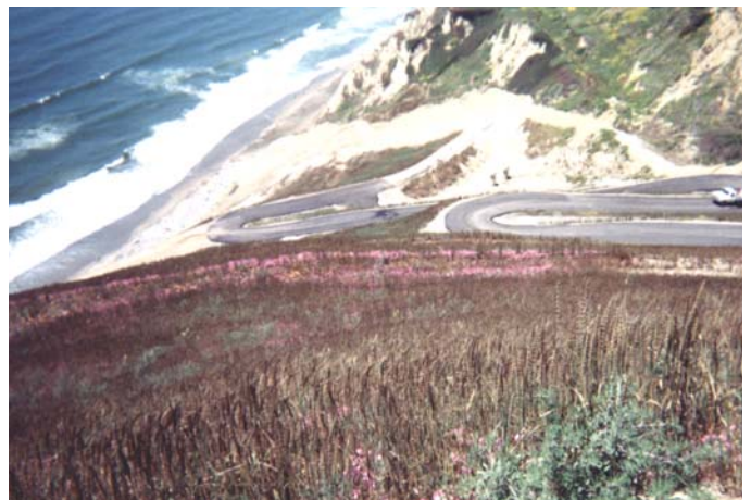
Avalon Canyon Slide Repair – July 1999 – Native Plant Establishment
